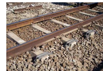
Installation of sleeper anchor in South Africa
